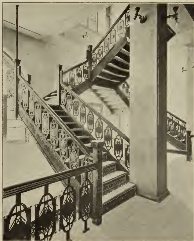
D.—STAIRWAY, UPPER FLOORS, CHICAGO STOCK EXCHANGE. Electroplated in Bronze. (Design by L. H. Sullivan.)
